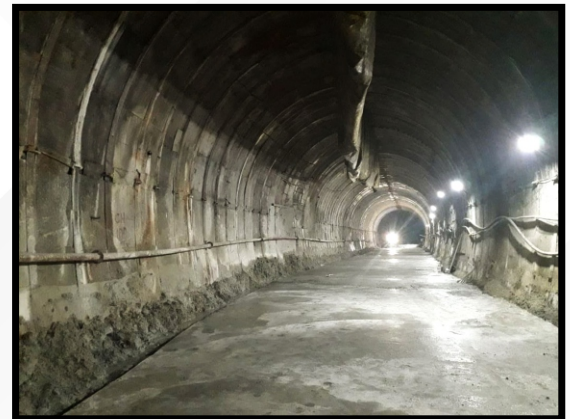
Rishikesh- Karnaprayag (new line) In Construction, RVNL
